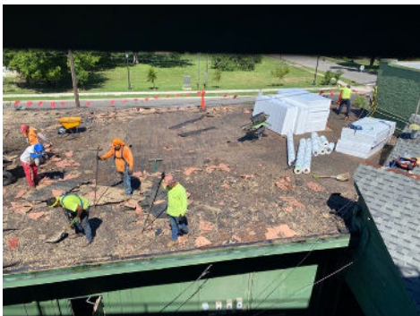
Rickwood’s Conference Room Roof ... Before
